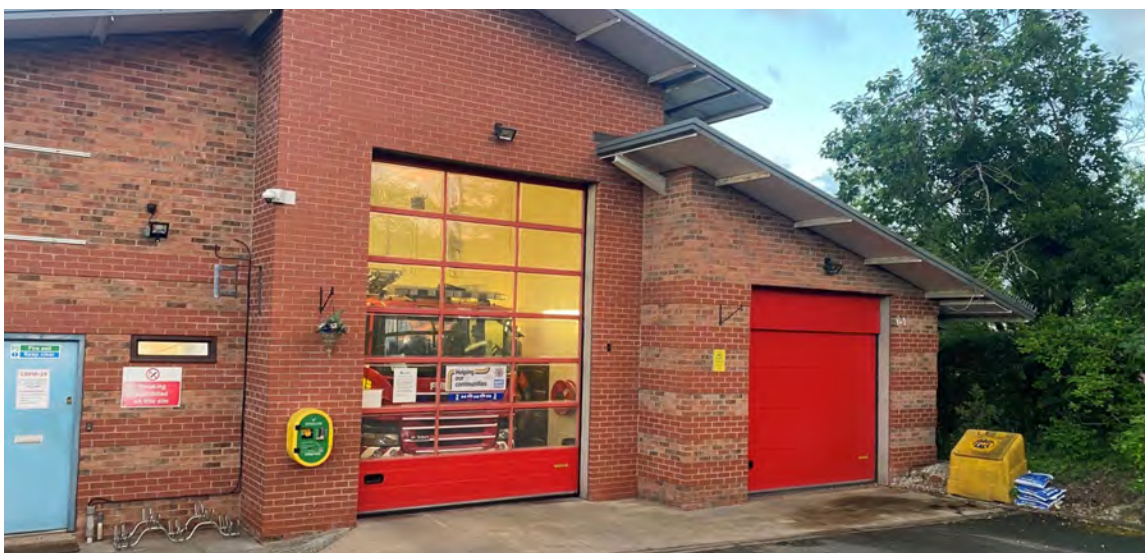
Malpas Fire Station
