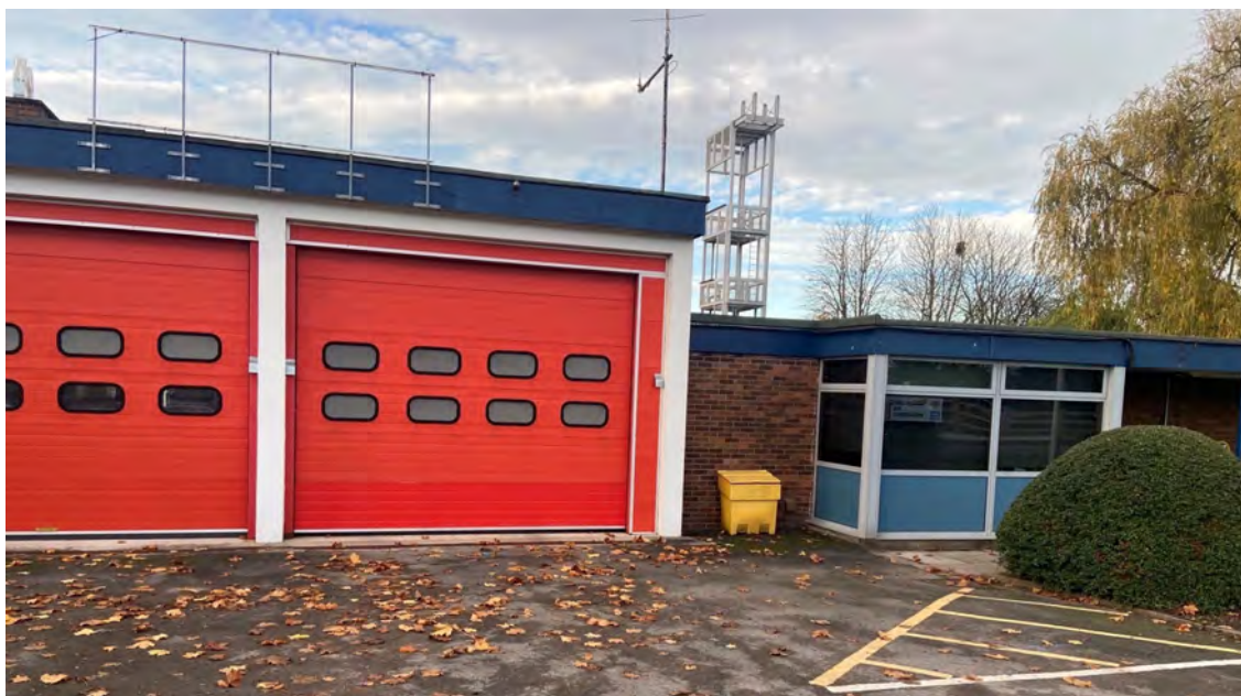
Knutsford Fire Station
